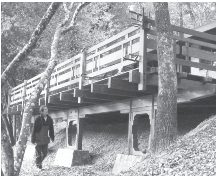
Figure 6. David inspecting a 60-foot deck rail made of Ipe, using Resorcinol urea resin glue.
